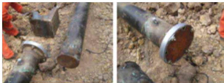
Figure N°38. Flange joint interim preparation
