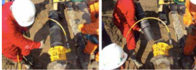
Figure 32. Placement of staples
