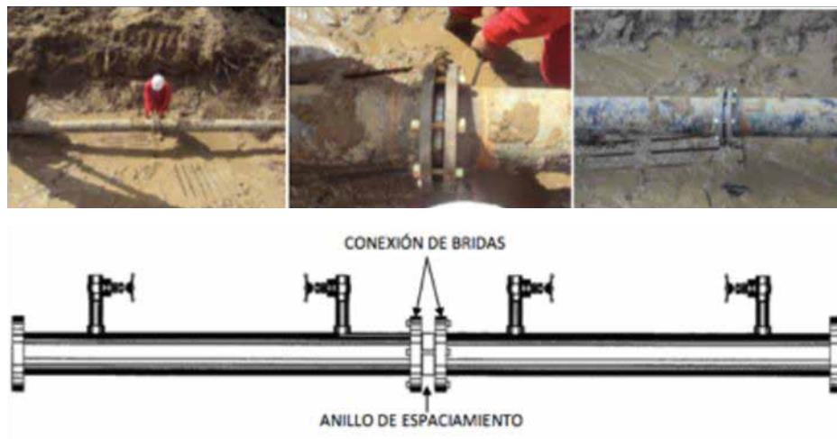
Figure N°35. Connecting the jacketed tube
