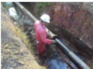
Figure N°24. Uniform bath to the polyethylene tube
