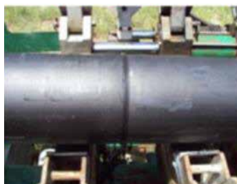
Figure N°16. Merging of pipelines
