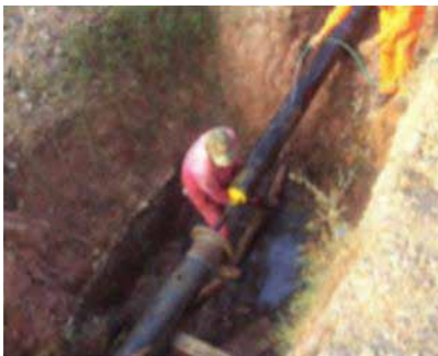
Figure N°23. Pulling the line through Dynawinch
