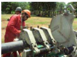
Figure N°25. Polyethylene Adjustment
