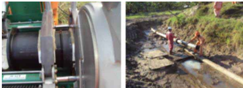
Figure 27. Cutting and thermofusion
